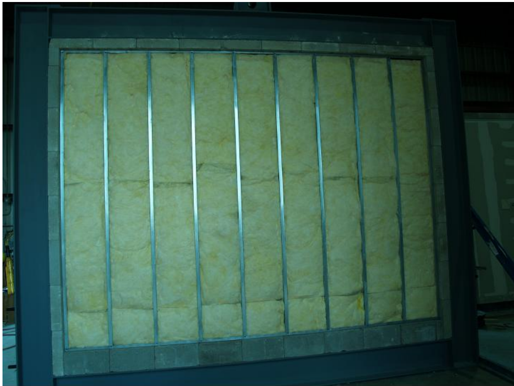
Figure B- 2. Test Wall during Construction.
