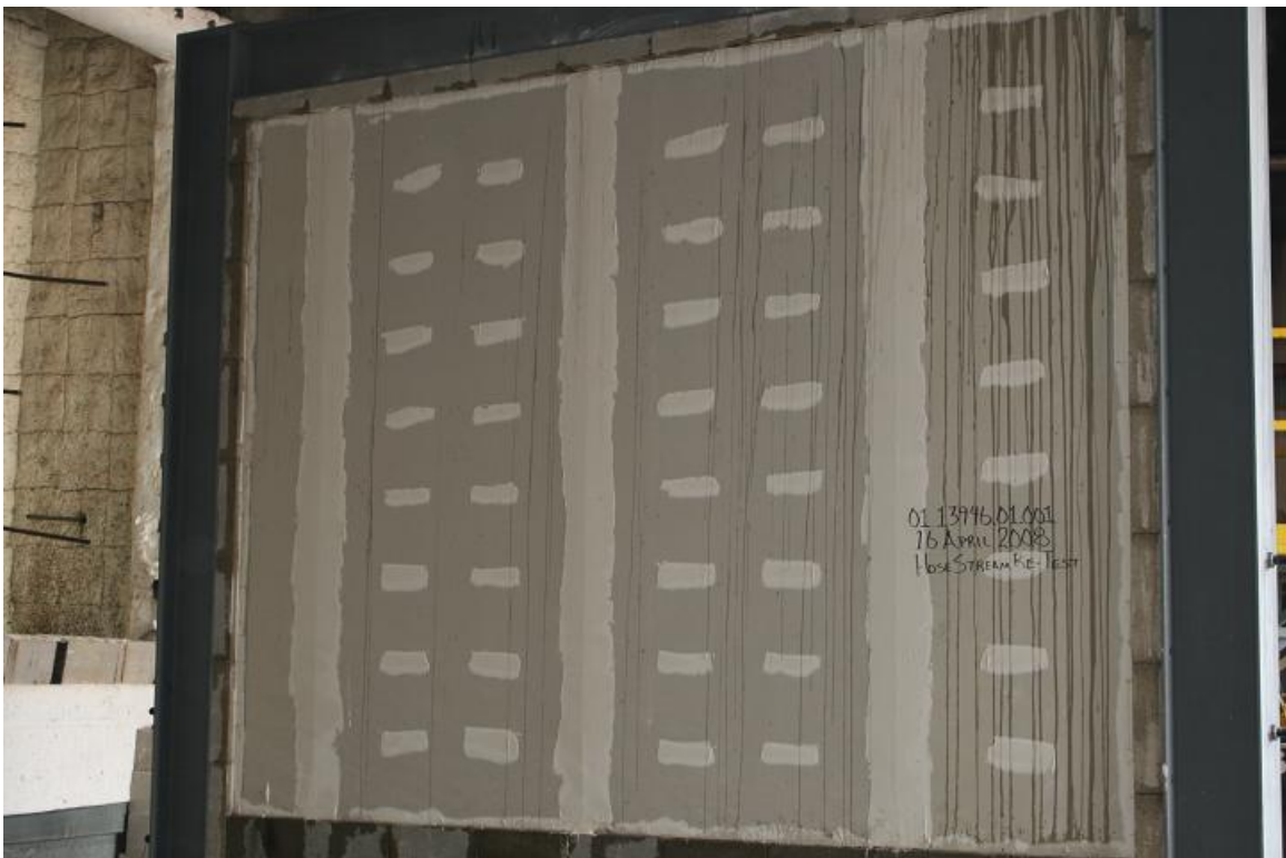
Figure B- 10. Unexposed Face after the Hose Stream Test.
