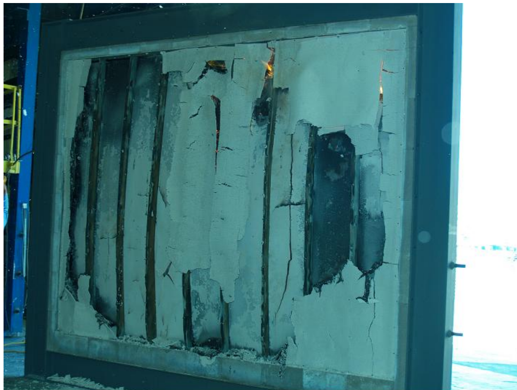
Figure B- 6. Exposed Face of Fire Test Wall at end of Furnace Exposure.
